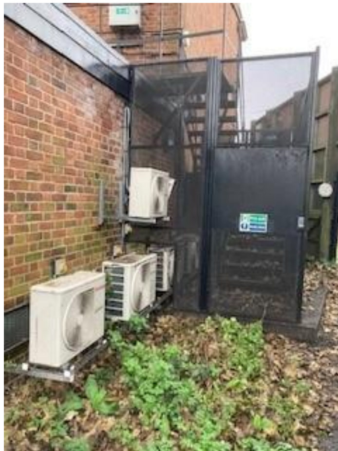
Adjacent Property's Security Cage at Rear of Site
